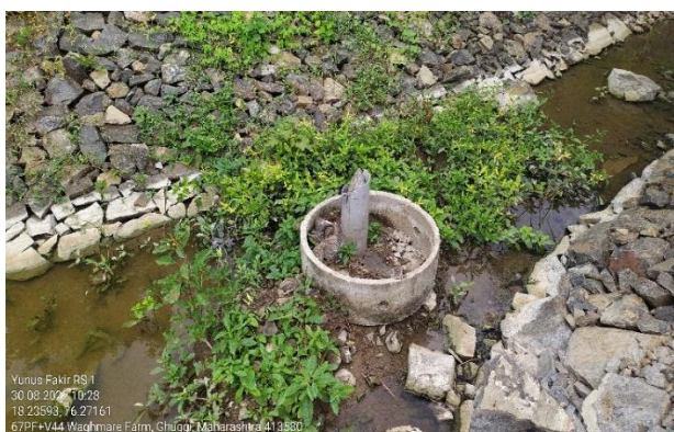
Damaged Cap and missing welded mesh of the recharge Hole in Ghuggi Village and siltation as well as debris of plants covering the structure
