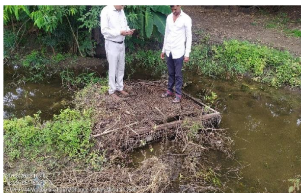
Damaged Cap and missing welded mesh of the recharge Hole in Ghuggi Village and siltation as well as debris of plants covering the structure
