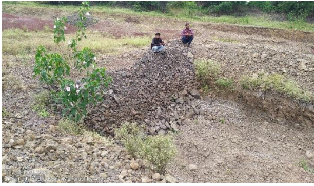
Stone pitching for the Recharge Shaft with Excavation
